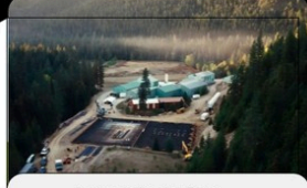
Antimony Smelter Plant – Thompson Falls, Montana Smelter capacity to expand to 300 tons per month or 11 tons per day
