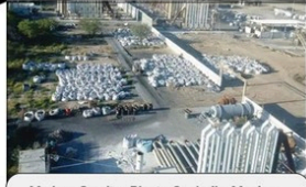
Madero Smelter Plant - Coahuila, Mexico Smelter capacity of 200 tons per month or 7 tons per day
